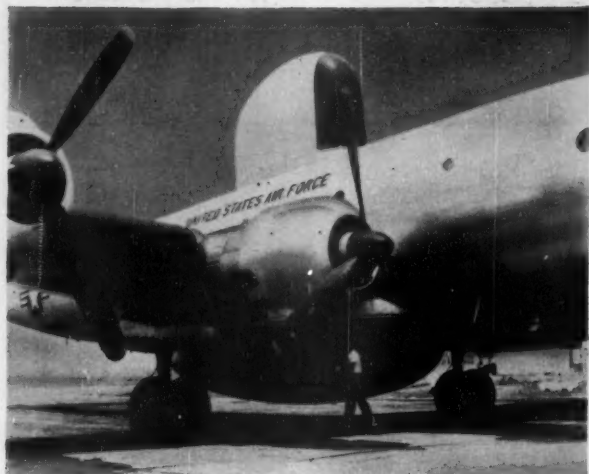
This flying radar station, with two tons of electronic equipment zippered into blister-like Radomes atop and below its fuselage, carries the world's most powerful airborne search radar. High-altitude planes with this system, twice as powerful as previous units, can search the upper air to provide early warning of sneak enemy air attacks.
